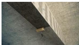
Applying epoxy resin
