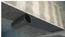
Pasting carbon fiber cloth
