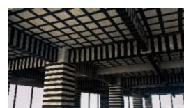
Curing and protecting
